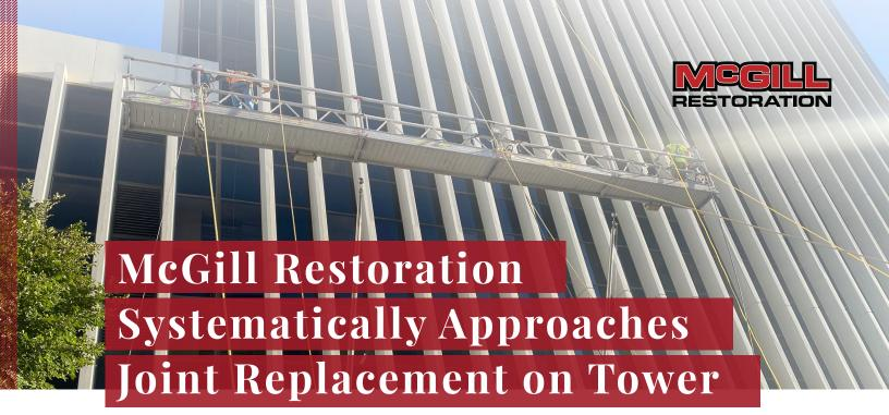
The U.S. Bank Tower is among the tallest buildings in downtown Lincoln, NE, and as such is a community landmark. Constant leaking created disruptions to tenants, ultimately forming a costly patchwork of temporary repairs. The building required a thorough approach to sealing joints with minimal tenant disturbance.
